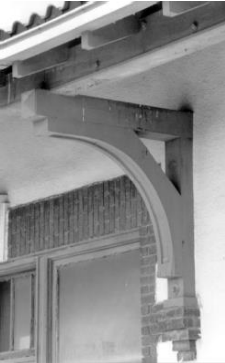
Exposed Rafters and Wood Bracket
