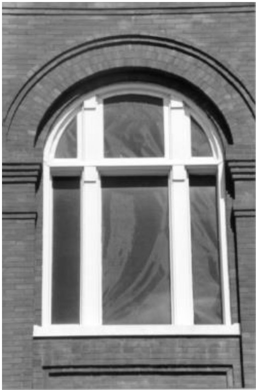
Arch with Fixed Infill Glazing
