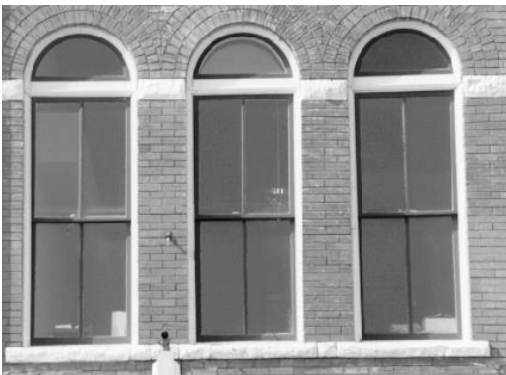
Round Arch, Fully Glazed over Hung Wood Sash, 2 over 2
