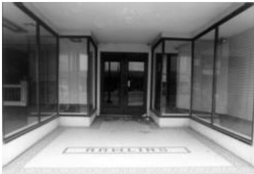
Recessed Bronze Storefront with Lettering in Mosaic Tile Floor
