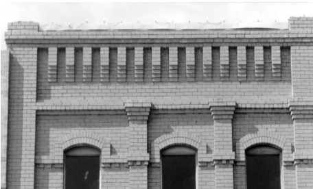
Brick Cornice and Articulated Segmental Arched Windows
