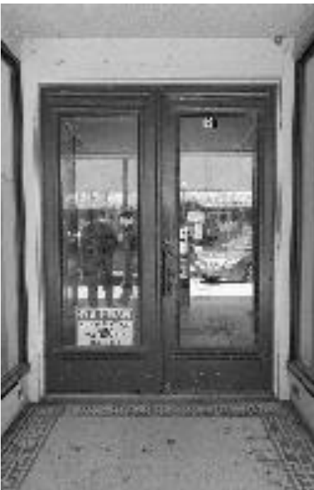
Wood Stile & Rail Doors with Original Mouldings
