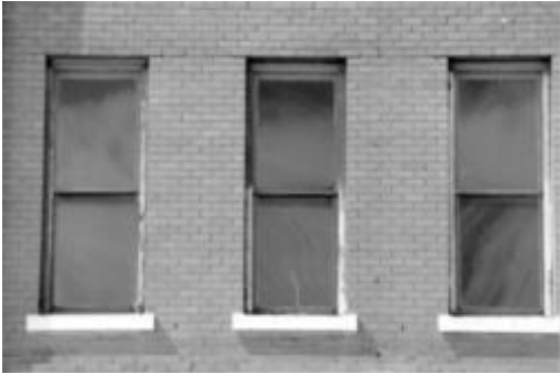
Rectangular, Fully Glazed Hung Wood Sash
