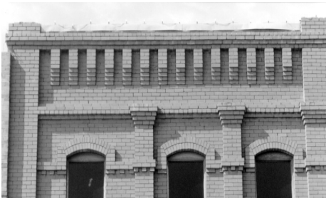
Brick Cornice and Articulated Segmental Arched Windows
