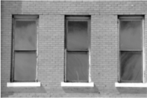
Rectangular, Fully Glazed Hung Wood Sash
