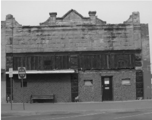
Before: Masonry and Wood Siding Infill in Traditional Locations for Glazed Clerestory and Storefront
