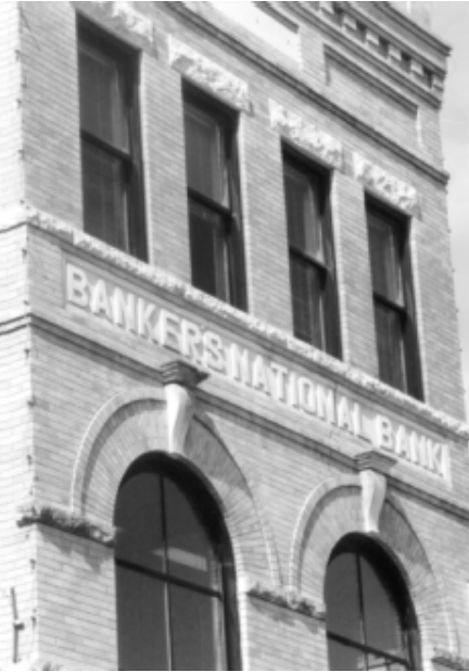
Brick Arches, Corbelled Cornice and Banding. Stone Lintels, Keys, Sills and Sign
