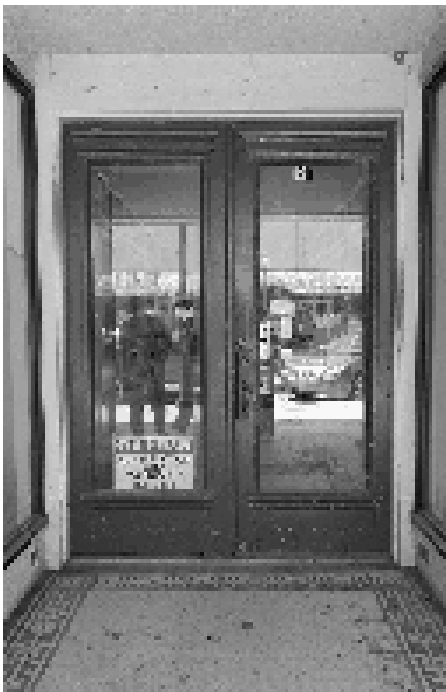
Wood Stile & Rail Doors with Original Mouldings
