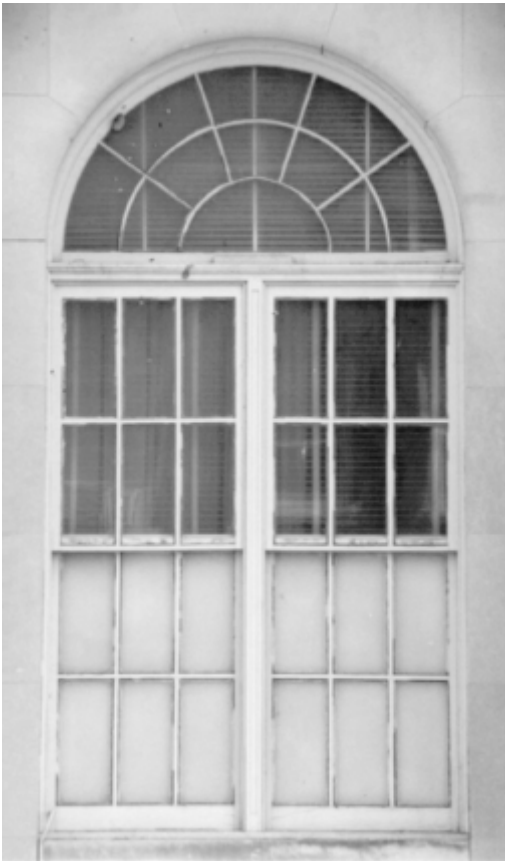
Divided Light Round Arch over Hung Wood Sash, 6 over 6
