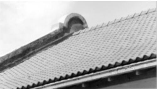
Tile Roof and Parapet Flashing with Exposed Cap
