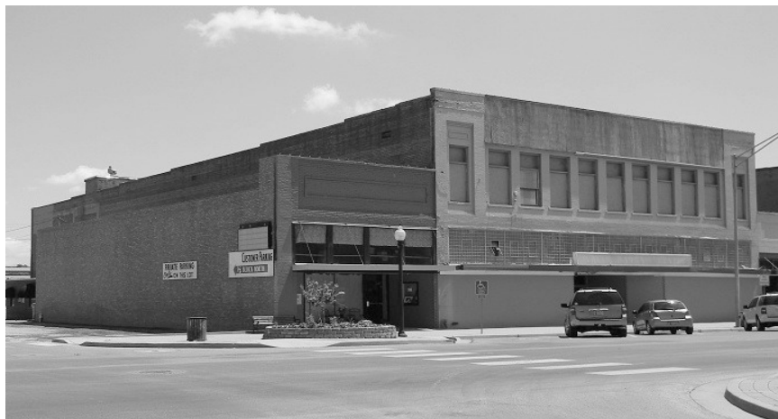
Stepped Parapet at Two Story Building Indicating Roof Slope
