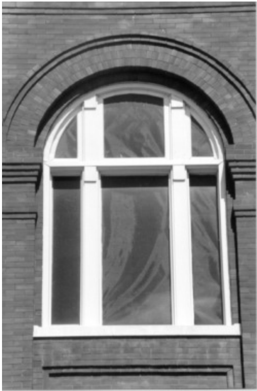
Arch with Fixed Infill Glazing
