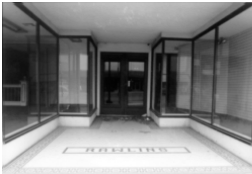
Recessed Bronze Storefront with Lettering in Mosaic Tile Floor
