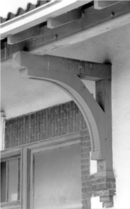
Exposed Rafters and Wood Bracket
