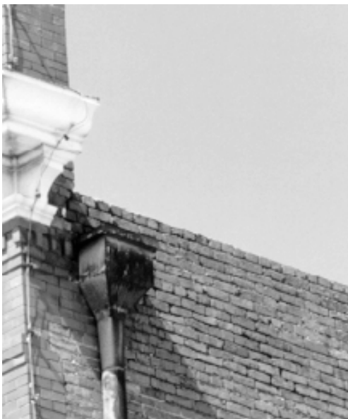
Parapet and Downspout
